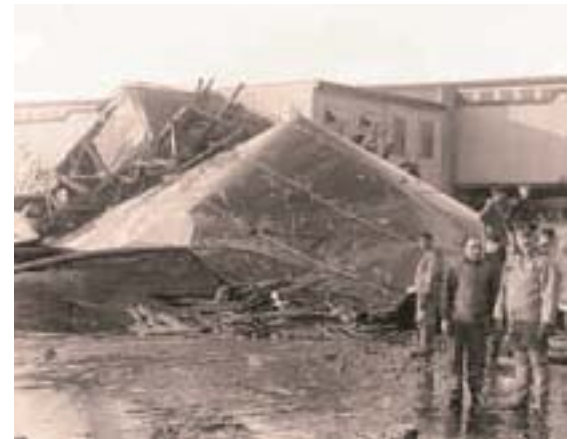
The molasses tank after the collapse
